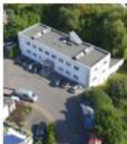
NOLDEN company site in Alfert near Bonn
